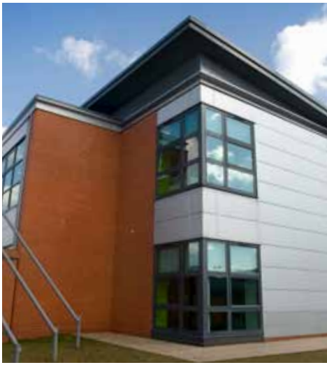
Self contained offices
